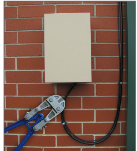
Even if an intruder cuts the exterior phone line, an alarm with radio backup installed will continue to function.
